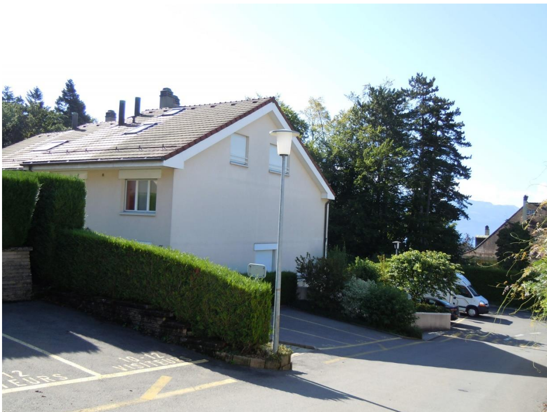
Residence of BATTISTOLO seen from the northwest
