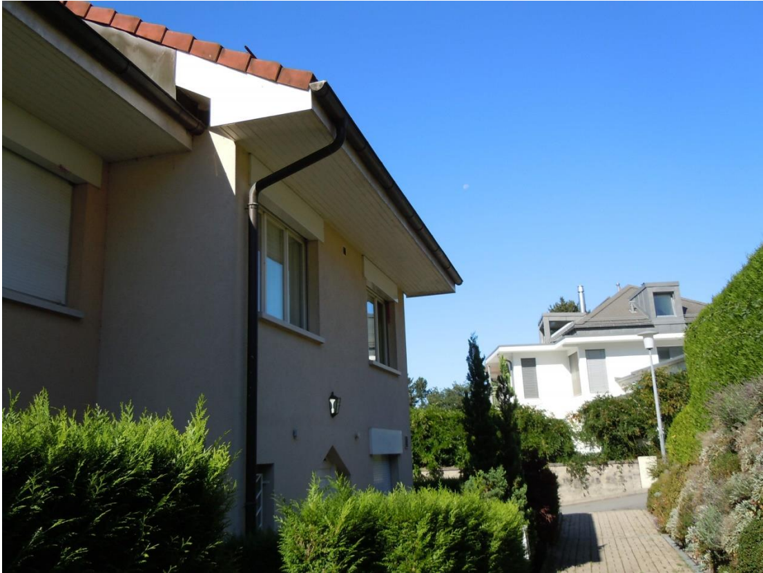
Residence of BATTISTOLO seen from the north side – entry (foreground)
