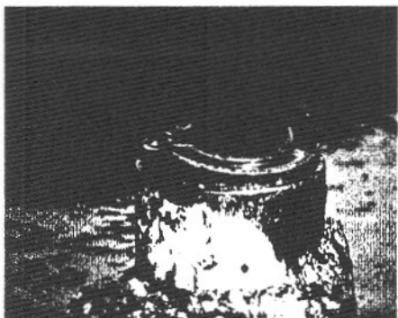
Fig. 1. The twin-nozzle abrasive jet cutter's primary advantage was its remote positioning and operating capabilities. This allowed wellhead equipment to be severed from burning wells and precluded the need for personnel to enter oil-flooded cellars (top photo). After cuts were made, wells were killed using stingers or capped using several different types of capping assemblies. Lower photo shows flow out of 7-in. casing that is being restricted by tubing, which fell downhole after being cut.
